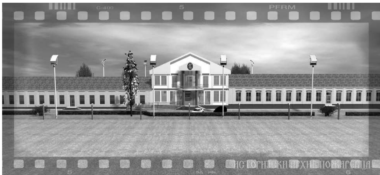
8. Jedinstveni (budući) arhivski kompleks Kasarna 4, vezni deo (nova zgrada) i kasarna 3 Istorijskog arhiva Požarevac 8. Unique (future) Archive complex Barracks 4, the connecting part (new building) and three barracks Historical Archives of Požarevac
